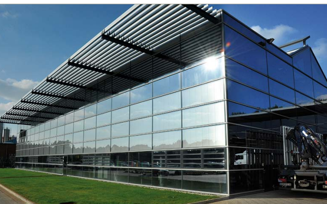
Left: The Glass Factory' which includes the sectors creaglas®, creacryl® and logistics, was opened in 2008.
